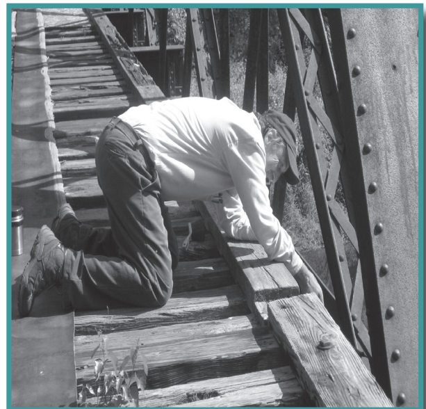
ABOVE: Bruce Peninno working on the lateral truss bridge.
